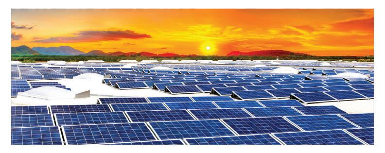
**Structural Considerations:** All rooftop solar projects undergo strict structural analysis before any project can commence. The average solar array weighs 3-4lbs per square foot. The average traditional hot tar and gravel roof weighs 7-10lbs. The True Seal system weighs as low as 0.47lbs per square foot including insulation, which makes this system an easy decision for any structural engineer.
